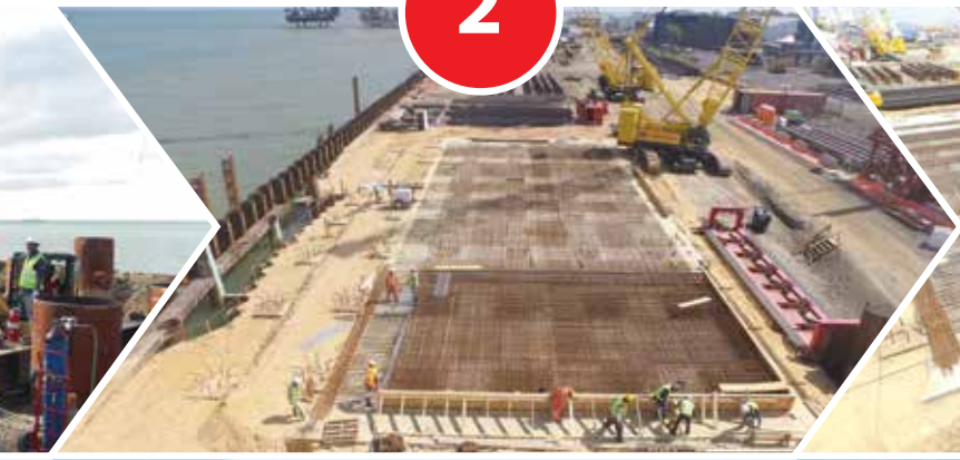
Installation of formwork for Phase 1 of HLP
