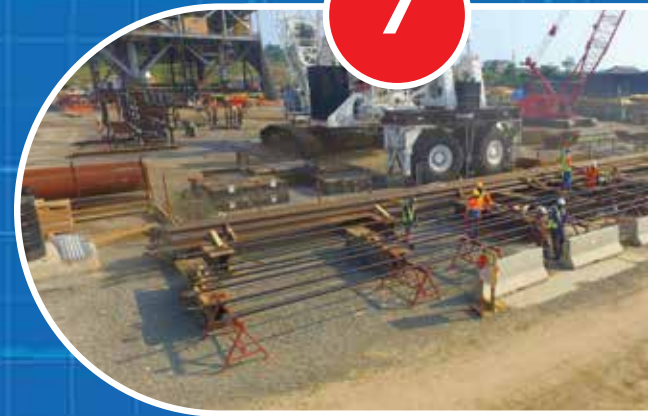
Tie rods are assembled in preparation for installation
