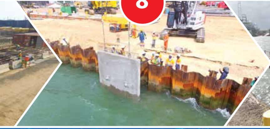
Precast fascia panels are installed at berth face
