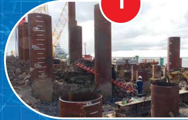
Tubular piles for new HLP are installed
