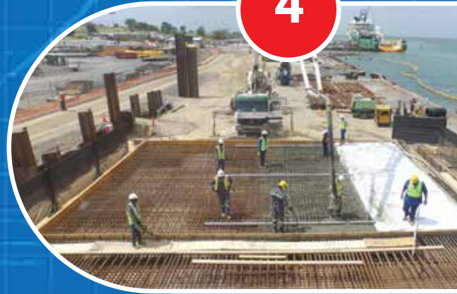
Concrete is poured for Phase 1 of HLP
