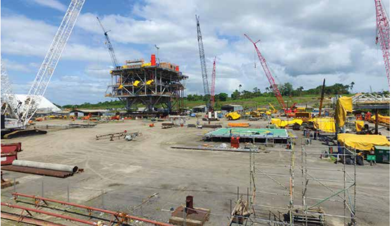
bpTT's Juniper Platform is constructed by TOFCO at Fabrication Yard, Port of Brighton
