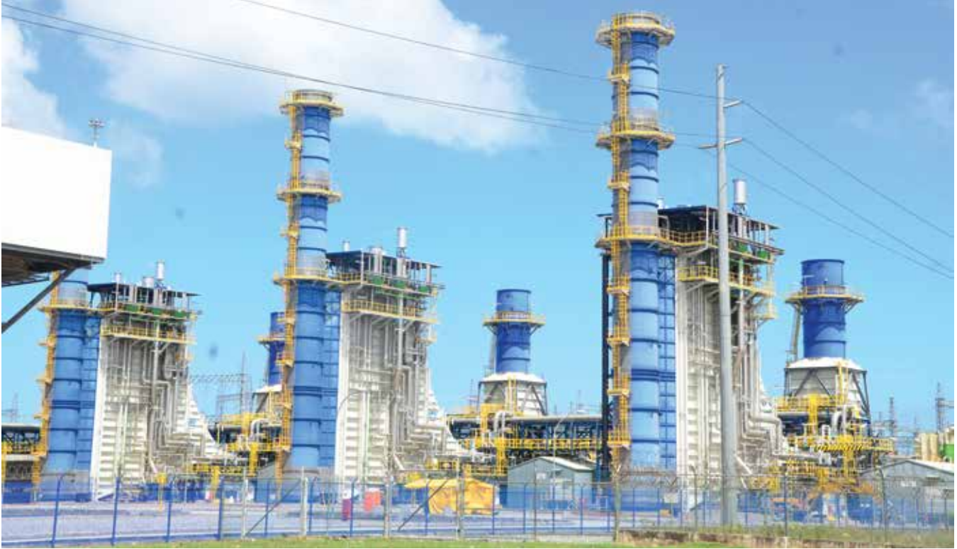
TGU Power Plant at Union Industrial Estate, La Brea
